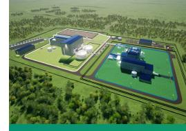
With the separation of major structures into a nuclear island and energy island, the Natrium plant requires less nuclear-grade safety equipment. It is designed to utilize construction material quantities that are comparable to a combined cycle plant and significantly less than other reactor designs.
